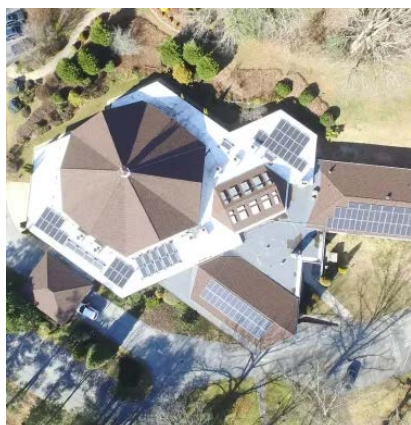
Trinity Presbyterian Church in Hendersonville, North Carolina, installed 129 solar panels in 2019, reducing its electricity consumption by 90% compared to the previous year. It's since become an Earth Care Congregation, promoting sustainability and environmental awareness. (Photo courtesy of Trinity Presbyterian Church)
